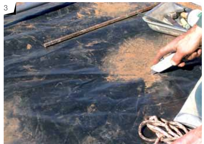
Photo 3: Cut hole in plastic.
