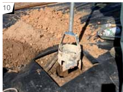
Photo 10: Augering to the next depth layer.
